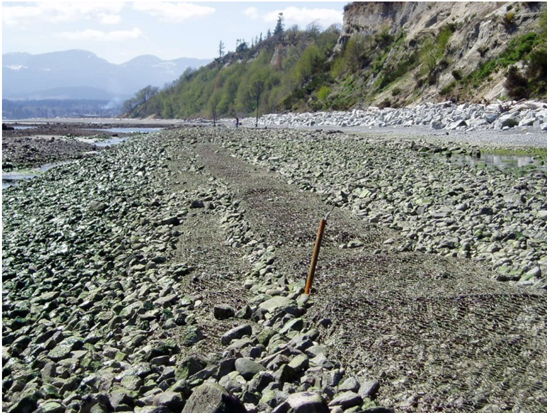
Photo 6: Waves have removed cobble-boulder cover and deposited material landward (April 2004)
